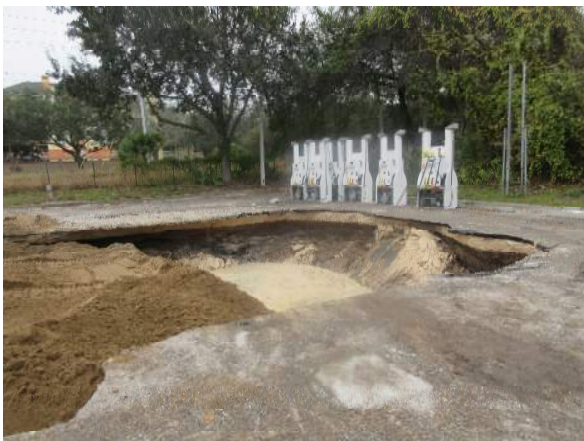
Photo #11 Partially backfilled tank excavation pit
