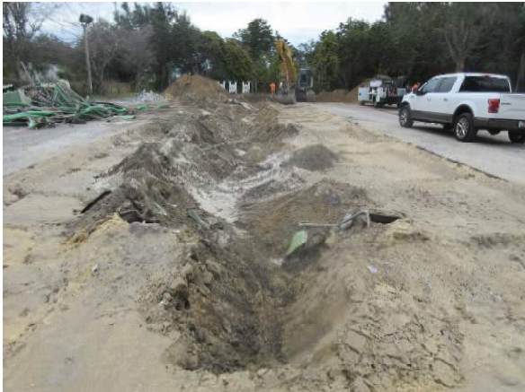
Photo #1 Fuel dispenser and fuel pipe line excavation toward the north
