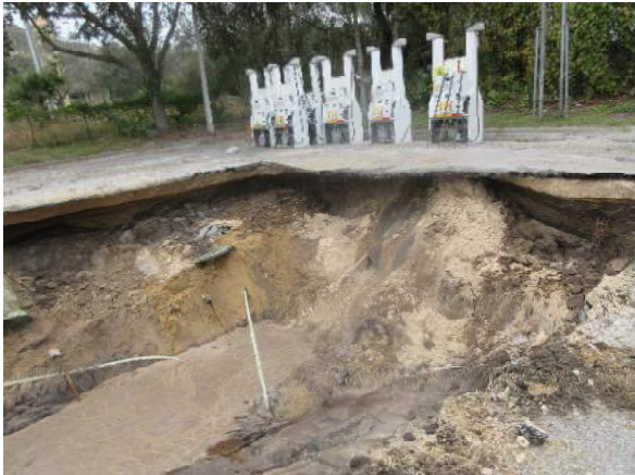
Photo #7 Northern side of the final tank excavation pit
