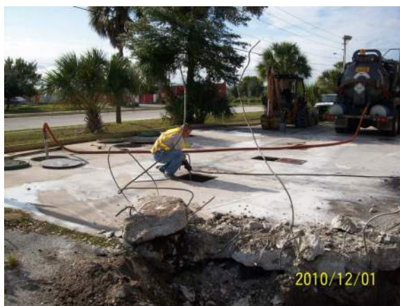
2010-12-02 USTs cleaned-pumped RMA
