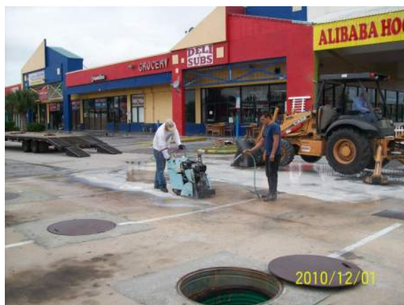
2010-12-01 Site prior to excavation RMA
