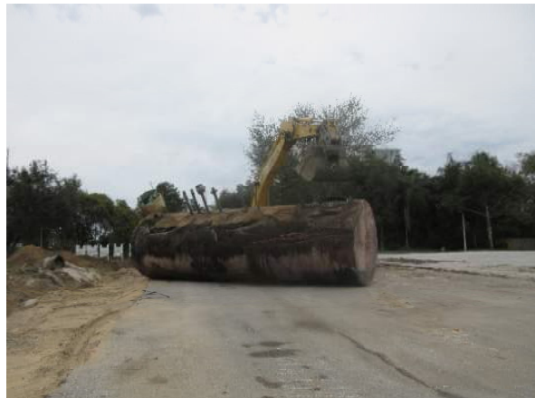
Photo #4 Excavated 20,000-gallon UST
