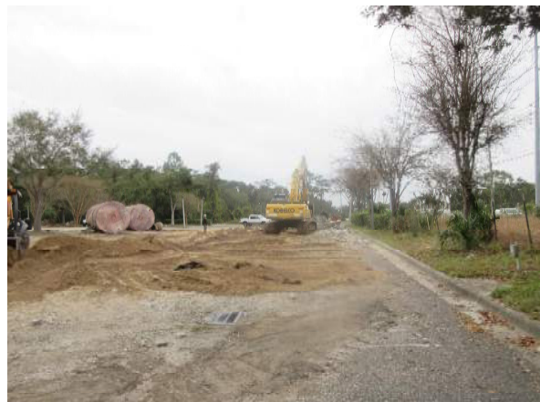
Photo #12 Excavated USTs and dispenser area
