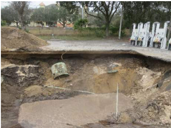
Photo #9 Western side of the final tank excavation pit
