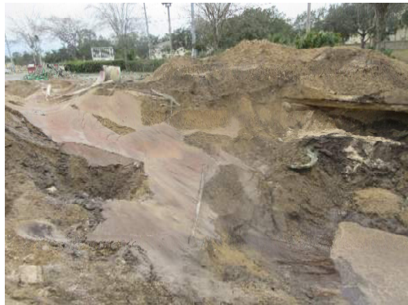
Photo #6 Southern side of the final tank excavation pit
