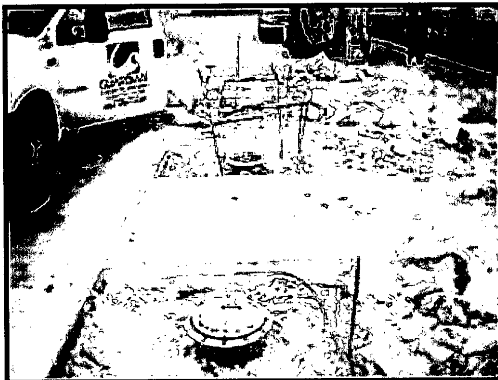
Hess 09267: Spill bucket replacement in progress on northern portion of property.
