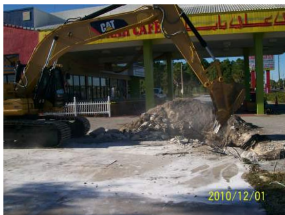
2010-12-01 Concrete removal RMA
