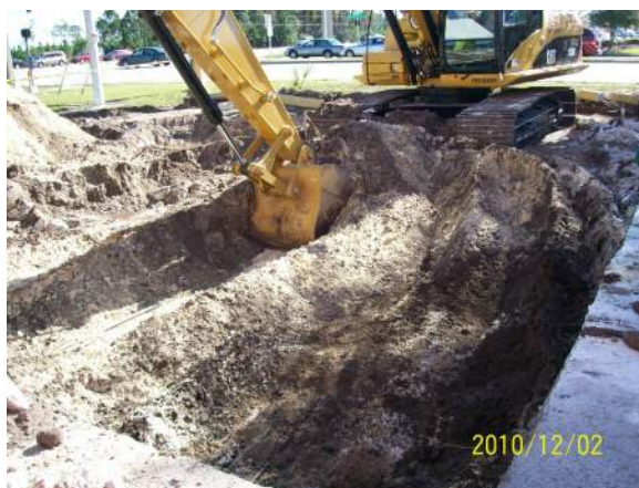
2010-12-02 Tank excavation RMA
