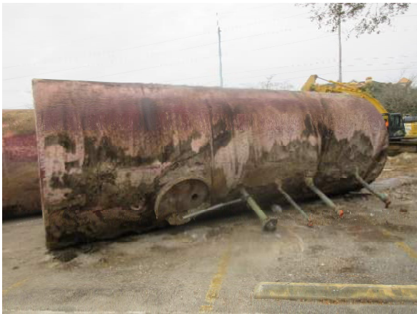
Photo #5 Excavated 16,000-gallon UST
