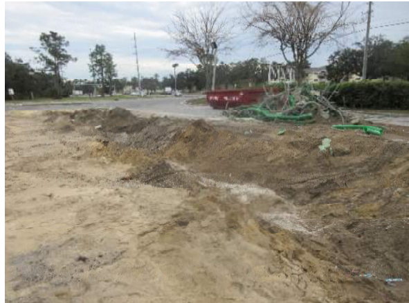
Photo #2 Fuel dispenser and fuel pipe line excavation toward the southwest
