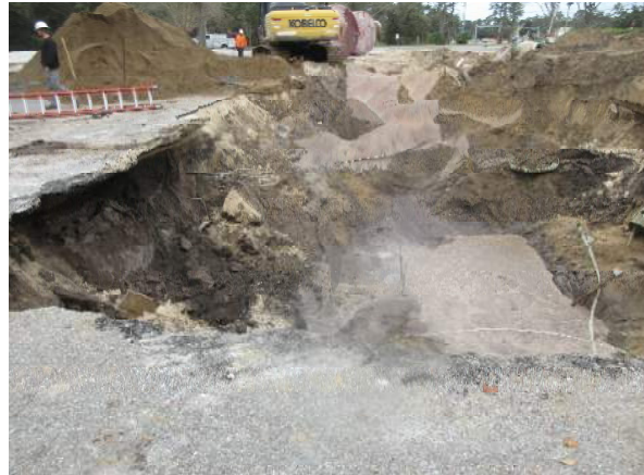
Photo #8 Eastern side of the final tank excavation pit
