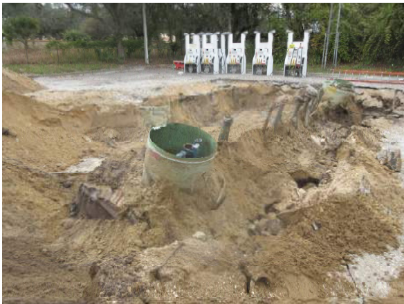
Photo #3 Partially excavated 20,000-gallon UST
