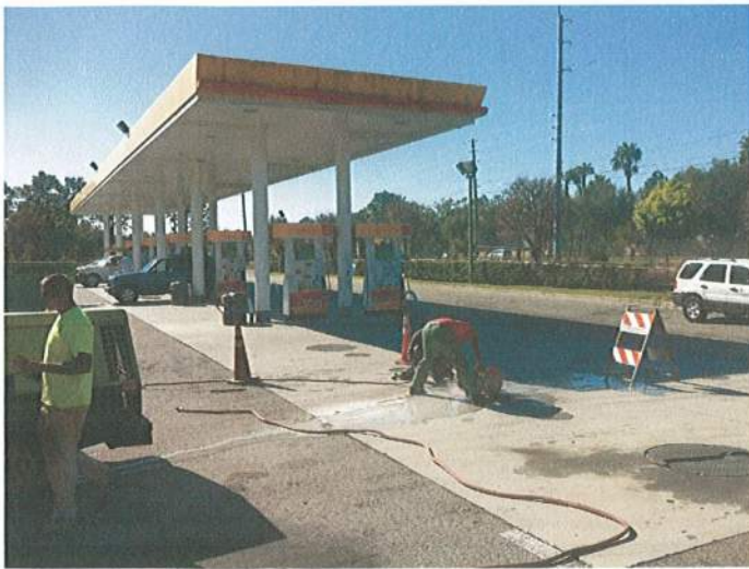
Photo 5: View of the removal the diesel spill bucket
