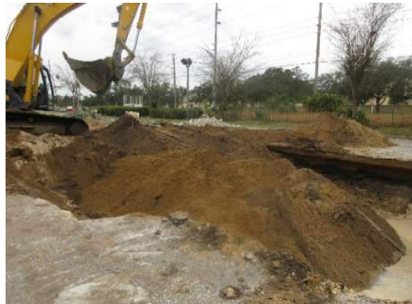
Photo #10 Backfill of the tank excavation with overburden soils
