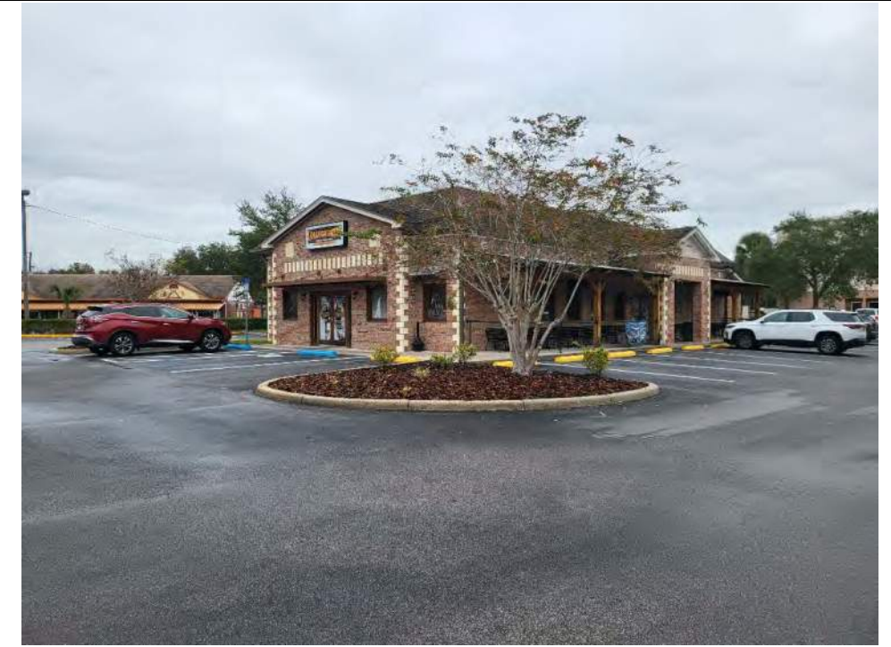
Looking northeast at the area of the former gas station location.
