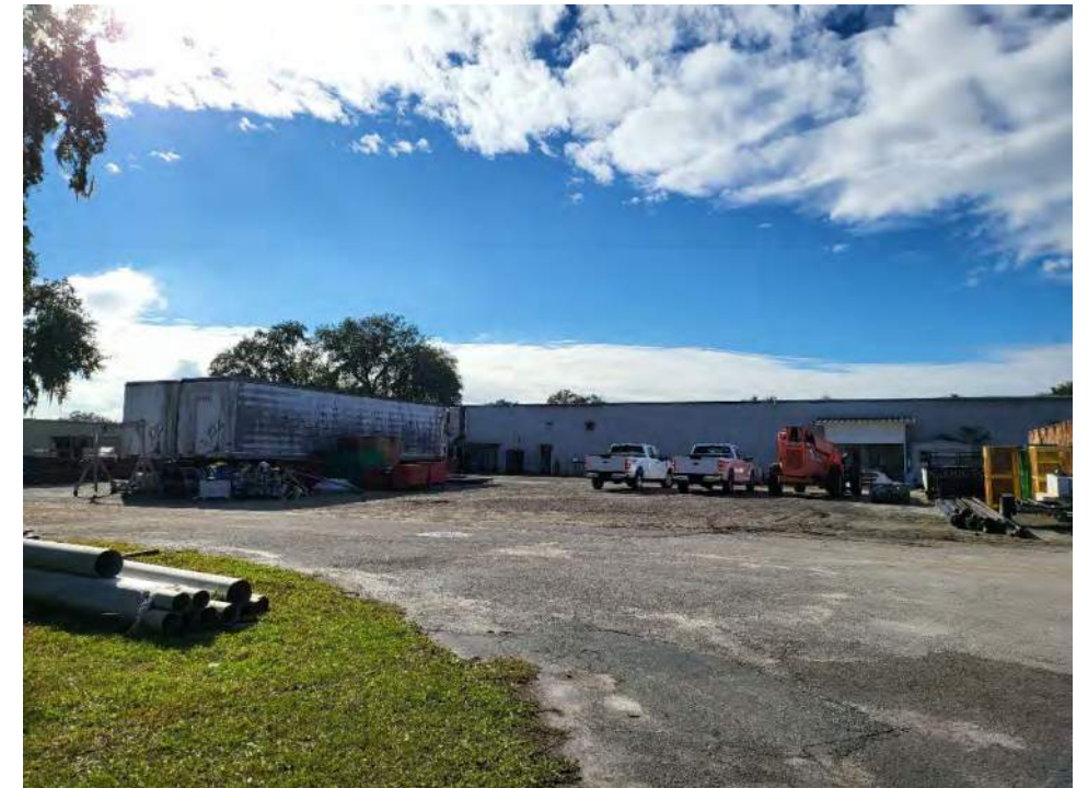
Looking west at the warehouse building.
