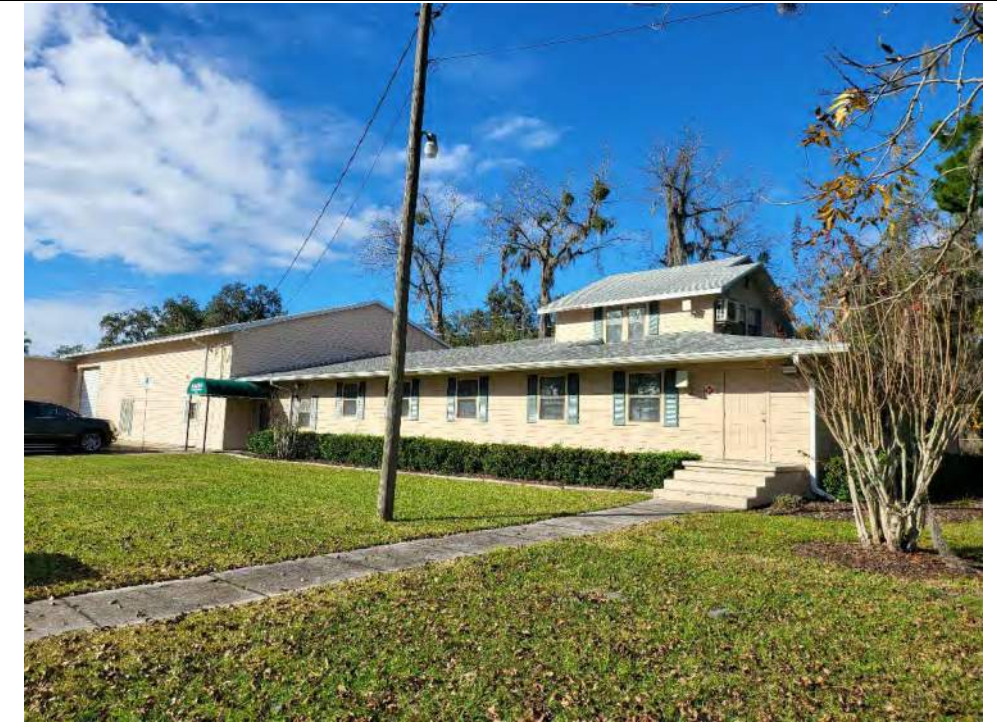
Looking northwest at the office building.
