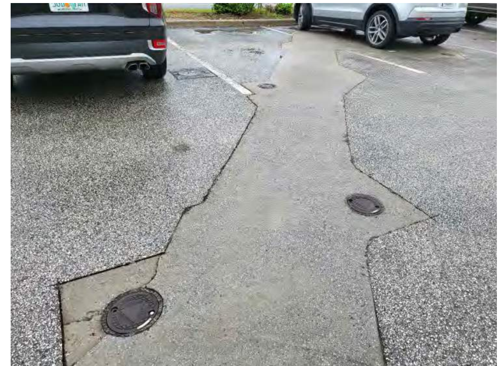
View of three remediation system wells in the eastern portion of the site.
