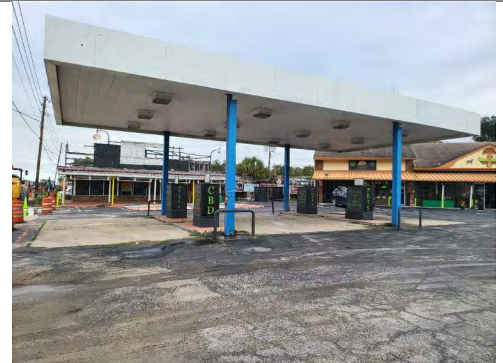
Looking north at the former fueling canopy.
