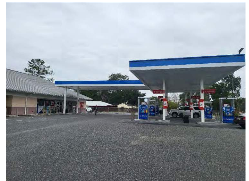
Looking north at the gas station and fueling pumps.
