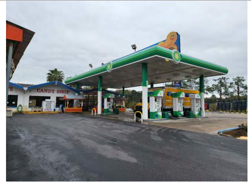
Looking east at the gas station and fueling pumps.
