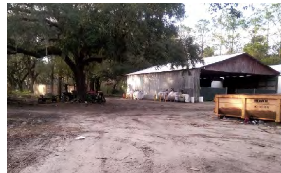
View of a maintenance garage and aboveground storage tanks.
