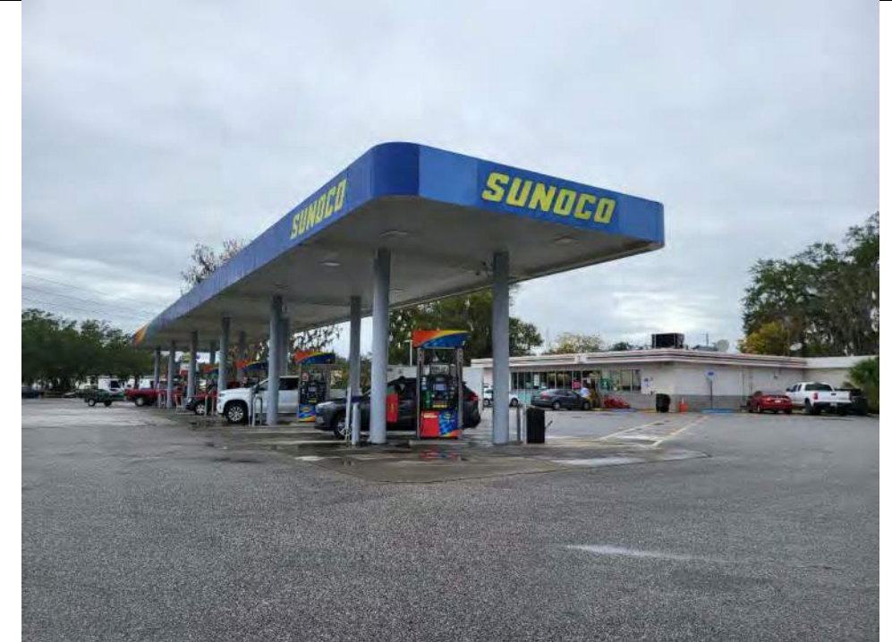
Looking northwest towards the gas station and fueling canopy.
