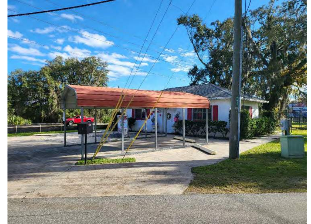
Looking south at the office building.
