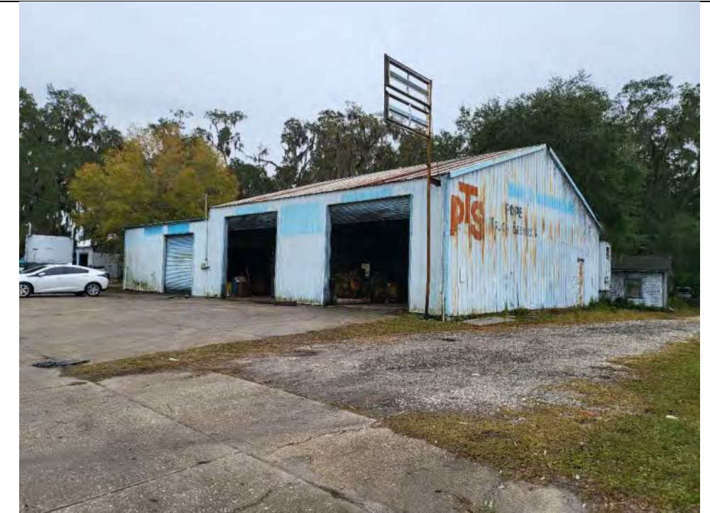
Looking southeast at the auto repair shop and potential former gas station.
