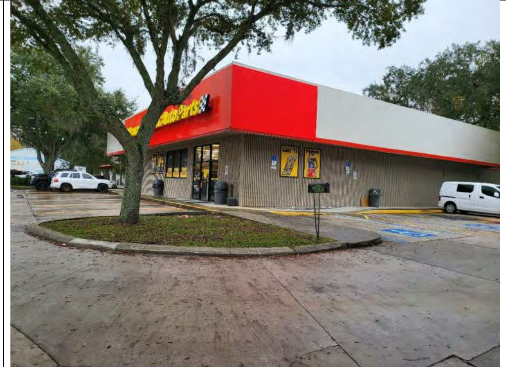
Looking southeast at the current retail building and area of the former gas station.
