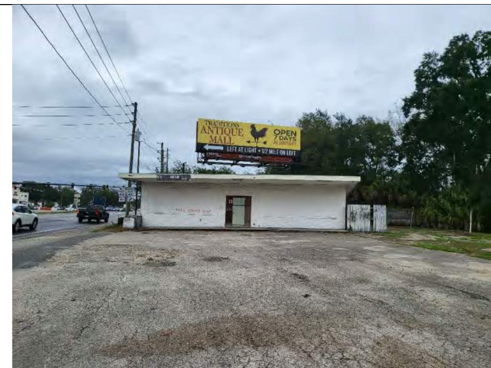
Looking north at the potential former gas station building.
