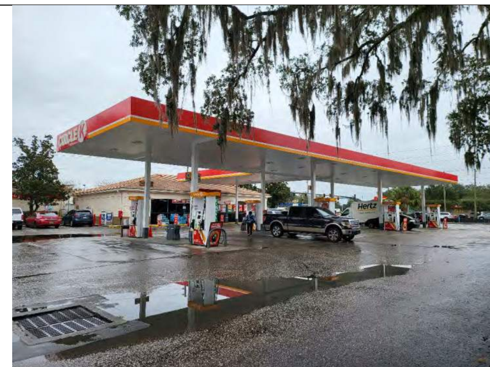
Looking northeast towards the gas station and fueling canopy.
