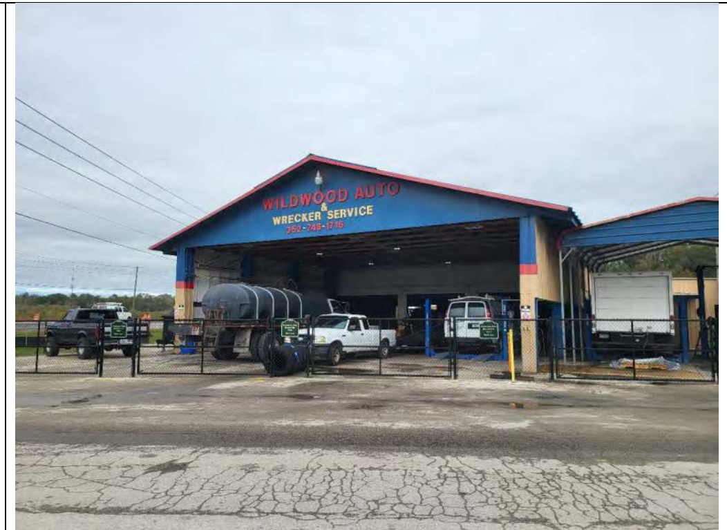
Looking north at the auto repair building.
