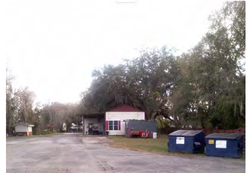
Looking south at the office building and a ~100-gallon aboveground storage tank.
