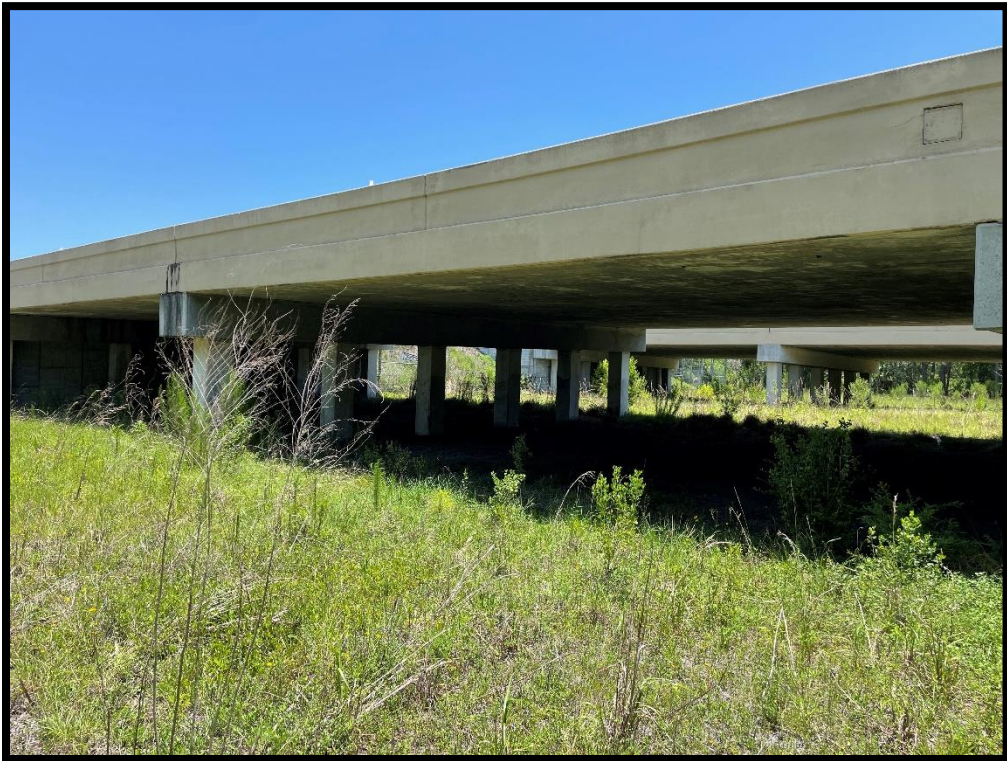
Photo 8: Wildlife crossing below I-4 located between Site 1A (eastbound) and Site 1B (westbound) truck parking areas
