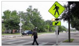
Rectangular Rapid Flashing Beacon
