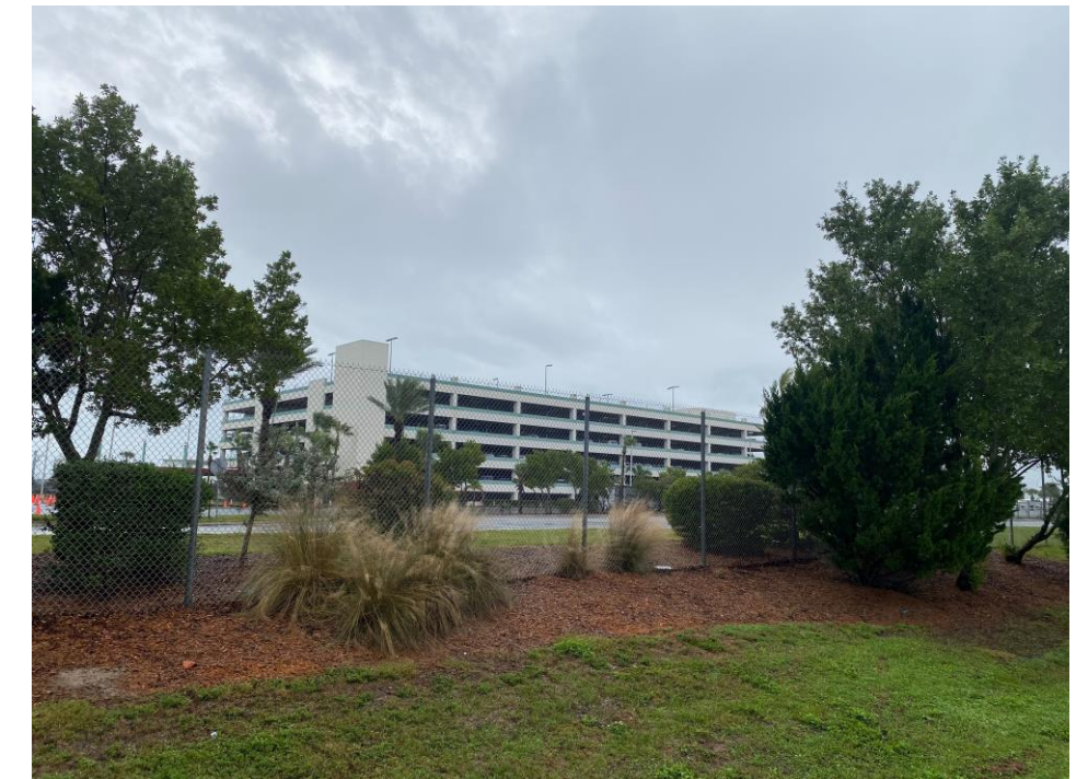
Looking east at the parking garage.
