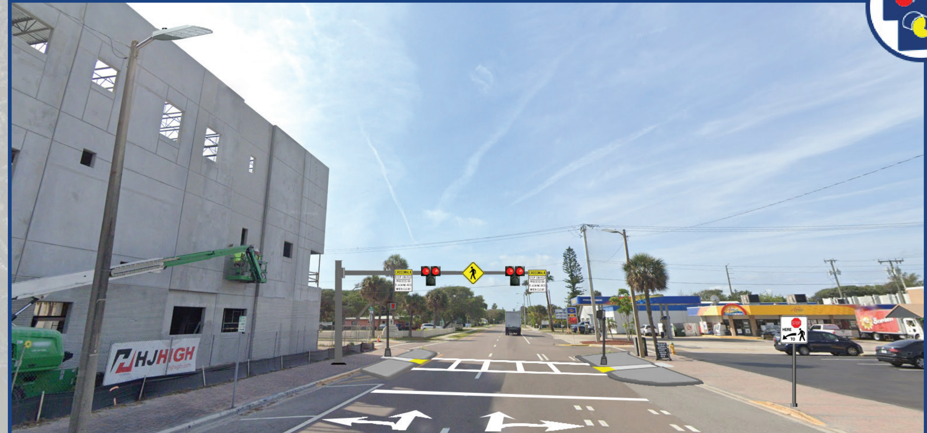
Example of Pedestrian Hybrid Beacon at 1 st St. S. (Southbound)
