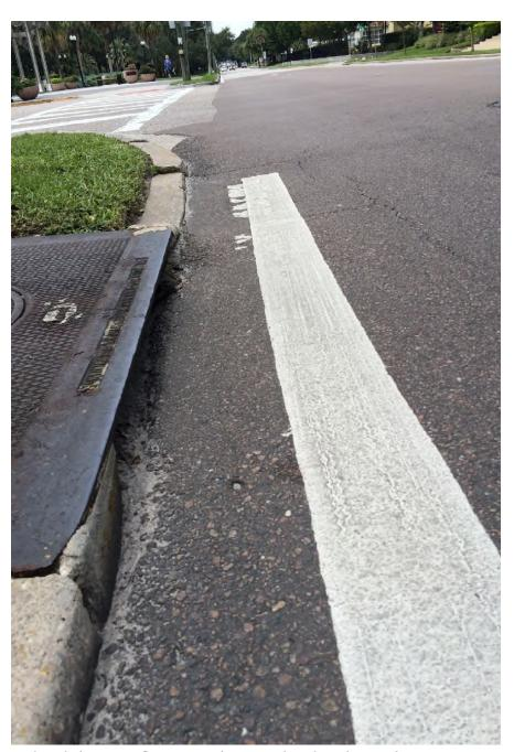
High asphalt restricts flow at some drainage inlets along the corridor.
