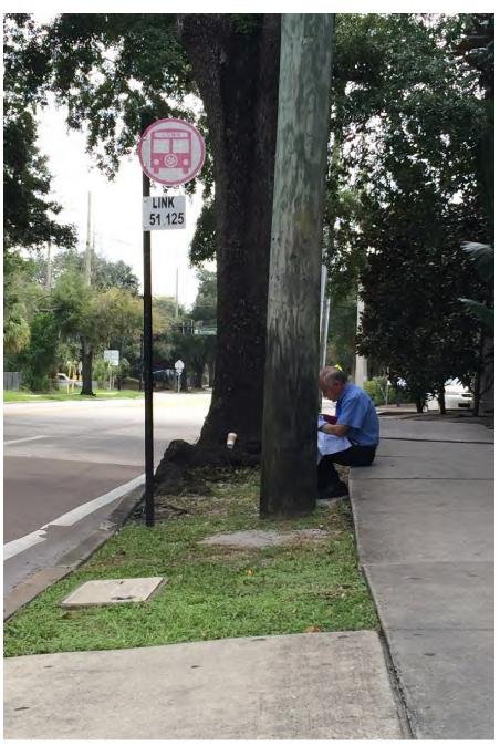
Tree roots cause curb line to shift and sidewalks to buckle at some locations.
