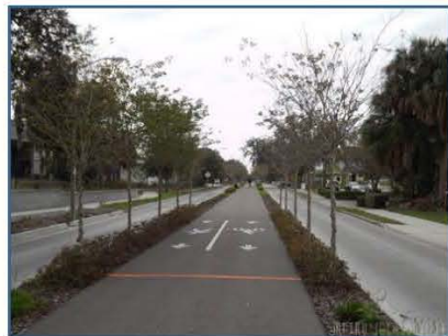
Cycle Track Pinellas Trail/Safford Avenue – Tarpon Springs
