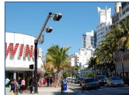
Widened Sidewalk SR A1A/Collins Avenue – Miami Beach
