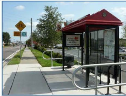
ADA Accessible Bus Stop SR 37/South Florida Avenue – Lakeland
