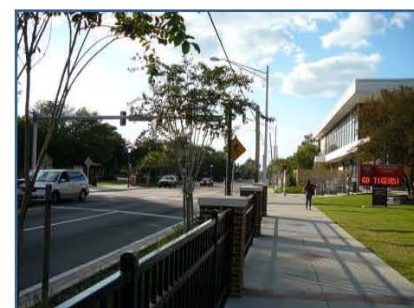
Pedestrian Channelization US 23/SR 139/Kings Road – Jacksonville
