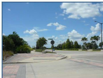
ADA Compliant Curb Lake Nona Boulevard – Orlando
