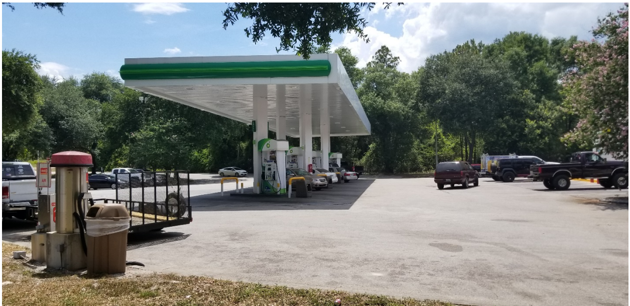
Photograph 6 Circle K Site 2 at intersection of Grand Ave. and W. New York Ave. (SR 44)
