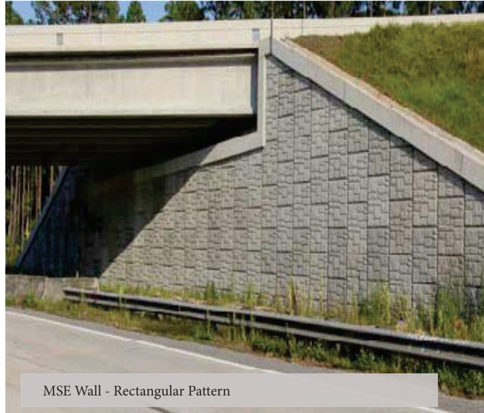
MSE Wall - Integrated with Traffic Barrier
