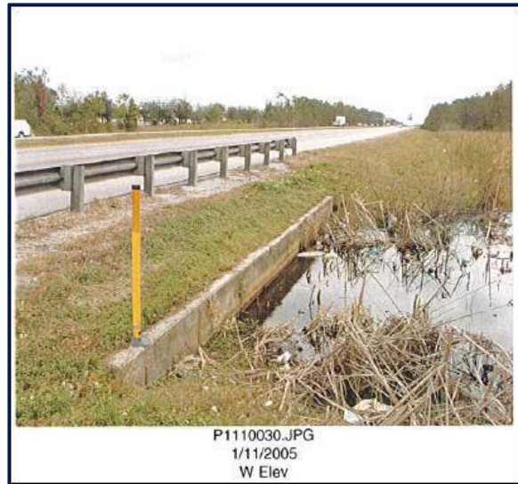
Figure 4 – High Water Condition, CD-4
