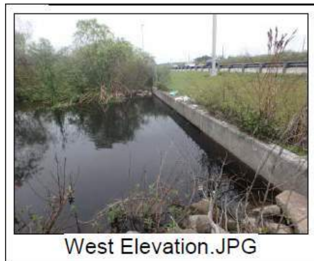
Figure 5 – High Water Condition, CD-5
